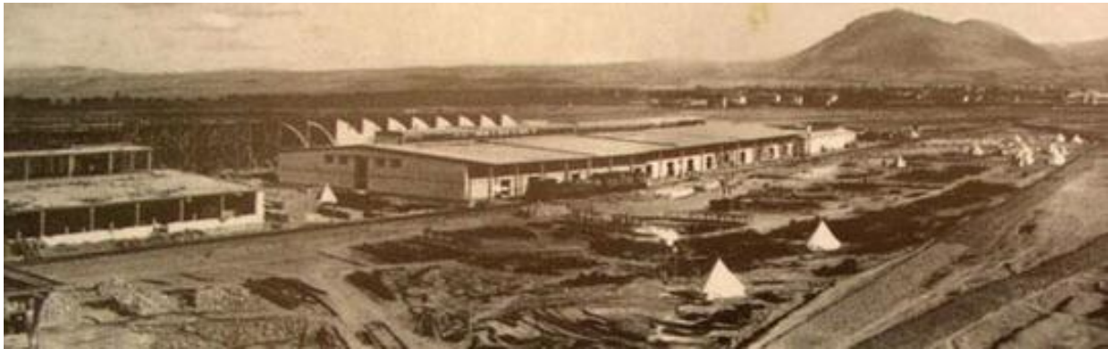
Picture 4: A photograph from the Factory Building (1934)
